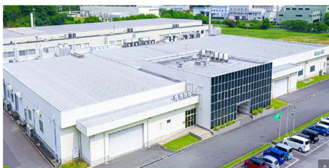
First and second HRDP lines at GEOMATEC's Ako Factory
