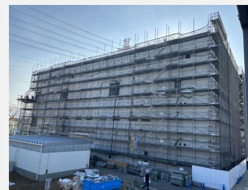
Initial mass production plant under construction
