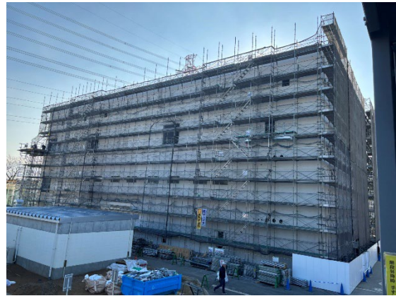
mass-production technology verification facility currently under construction
