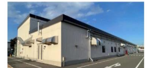
A-SOLiD® mass production testing building (Ageo City)
