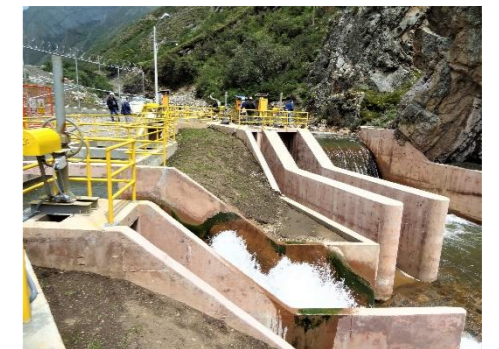
Water intake of the hydroelectric power plant (near the Pallca Mine)
