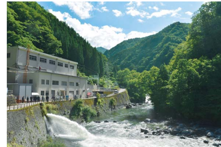
Kanakido power plant, Kamioka Mining and Smelting Co., Ltd.
