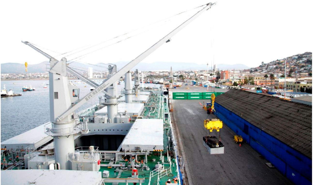
Photo: Loading the initial shipment of Caserones copper concentrate onto the Koryu carrier ship
