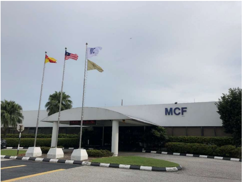
Mitsui Kinzoku Plant in Malaysia (Mitsui Copper Foil (Malaysia) SDN. BHD.)
